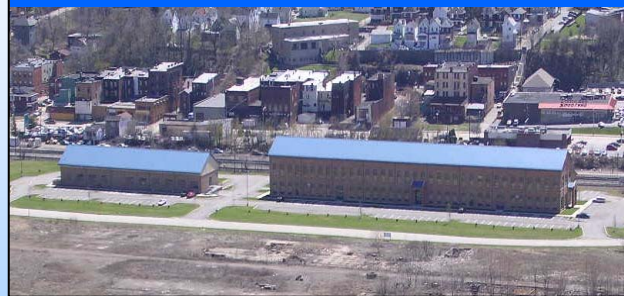
MAGLEV, Inc. R&D Facility in McKeesport, PA
