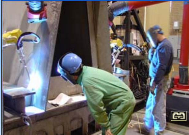
Dual Robot Synchronous Welding of Model Beam
